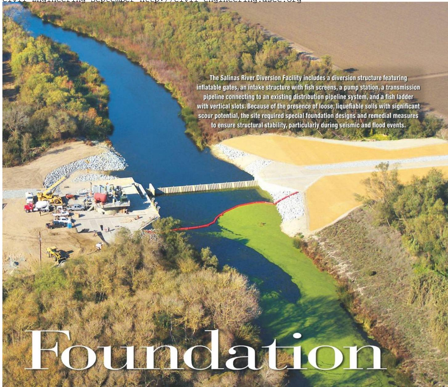
The Salinas River Diversion Facility includes a diversion structure featuring inflatable gates, an intake structure with fish screens, a pump station, a transmission pipeline connecting to an existing distribution pipeline system, and a fish ladder with vertical slots. Because of the presence of loose, liquefiable soils with significant scour potential, the site required special foundation designs and remedial measures to ensure structural stability, particularly during seismic and flood events.
