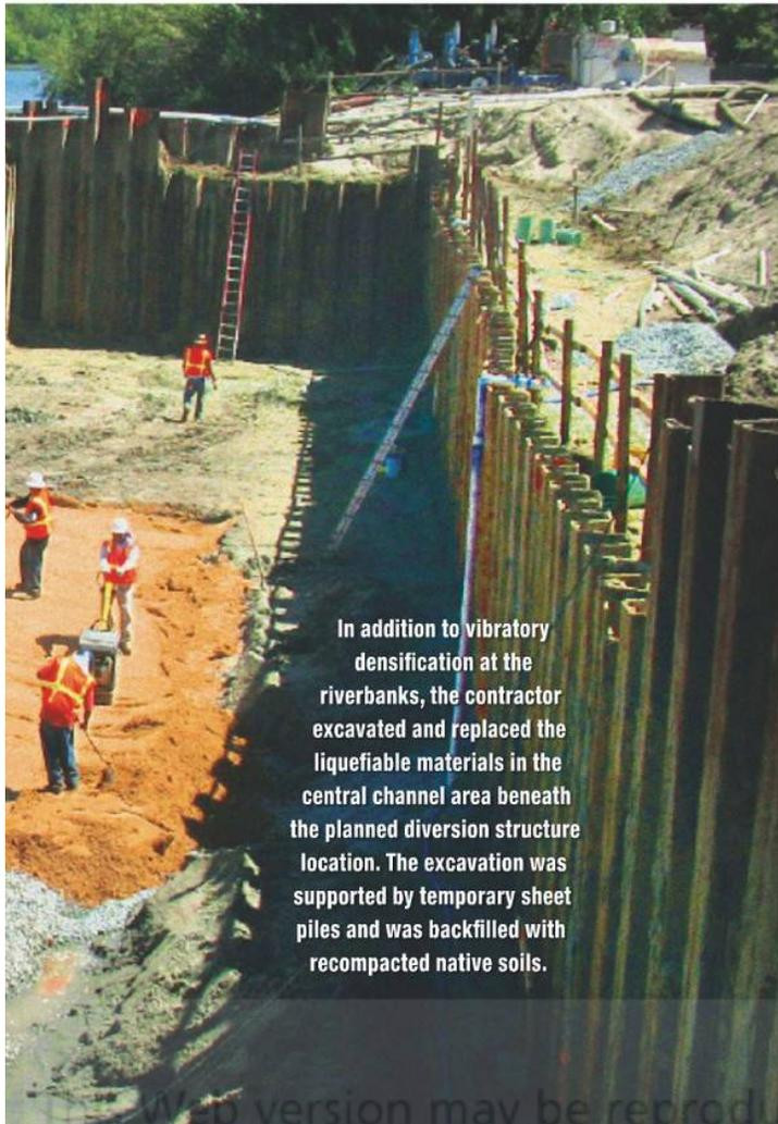
In addition to vibratory densification at the riverbanks, the contractor excavated and replaced the liquefiable materials in the central channel area beneath the planned diversion structure location. The excavation was supported by temporary sheet piles and was backfilled with recompacted native soils.
